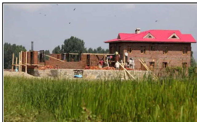
Fig. 1 : Construction of a house in the paddy field
